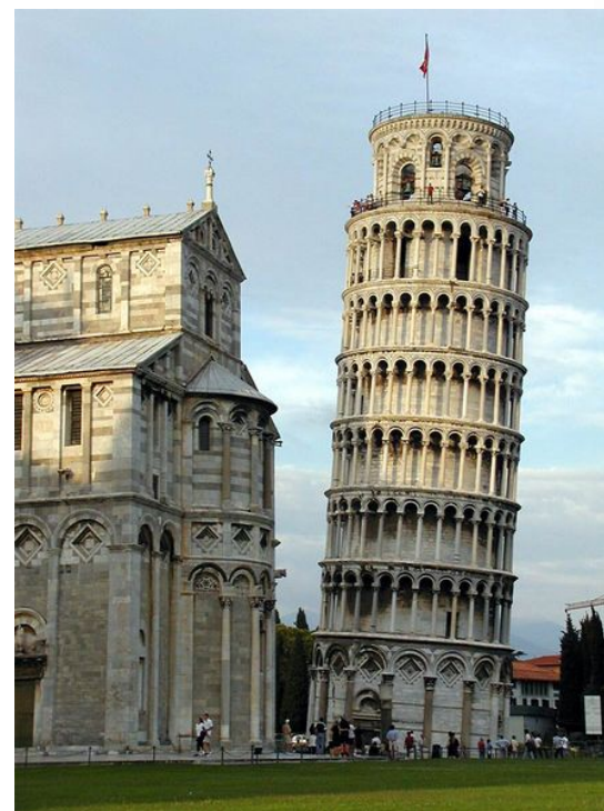
Example of bad practice
